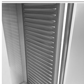
Internal details of deep-drawn stainless steel-sides
