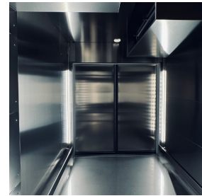
LED internal lighting
