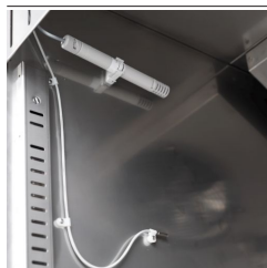
Humidity control with electronic probe
