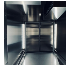
Internal lighting with LED lights
